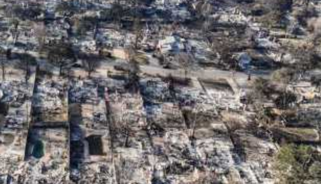
Entire Neighborhood destroyed by the Eaton Fire
